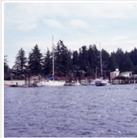
Manson's Landing wharf, view from the water
