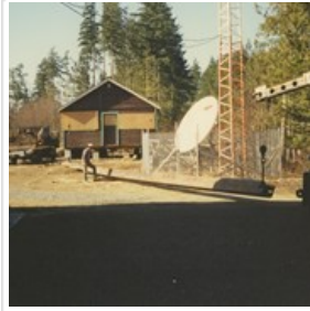
Moving the museum: steel beam supports being removed ...
